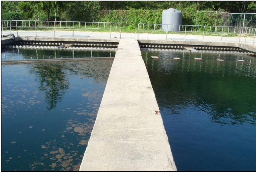
Sedimentation Basin (Left Side)–Renovated MIDAF system (Right Side) Renovated MIDAF system (Left Side)–Sedimentation Basin (Right Side)
